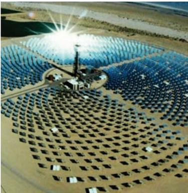
Solar Two Project, developed by Bechtel, was a 10 MW Concentrated Thermal Solar Power Plant, with a molten salt system, in California's Mojave Desert.
