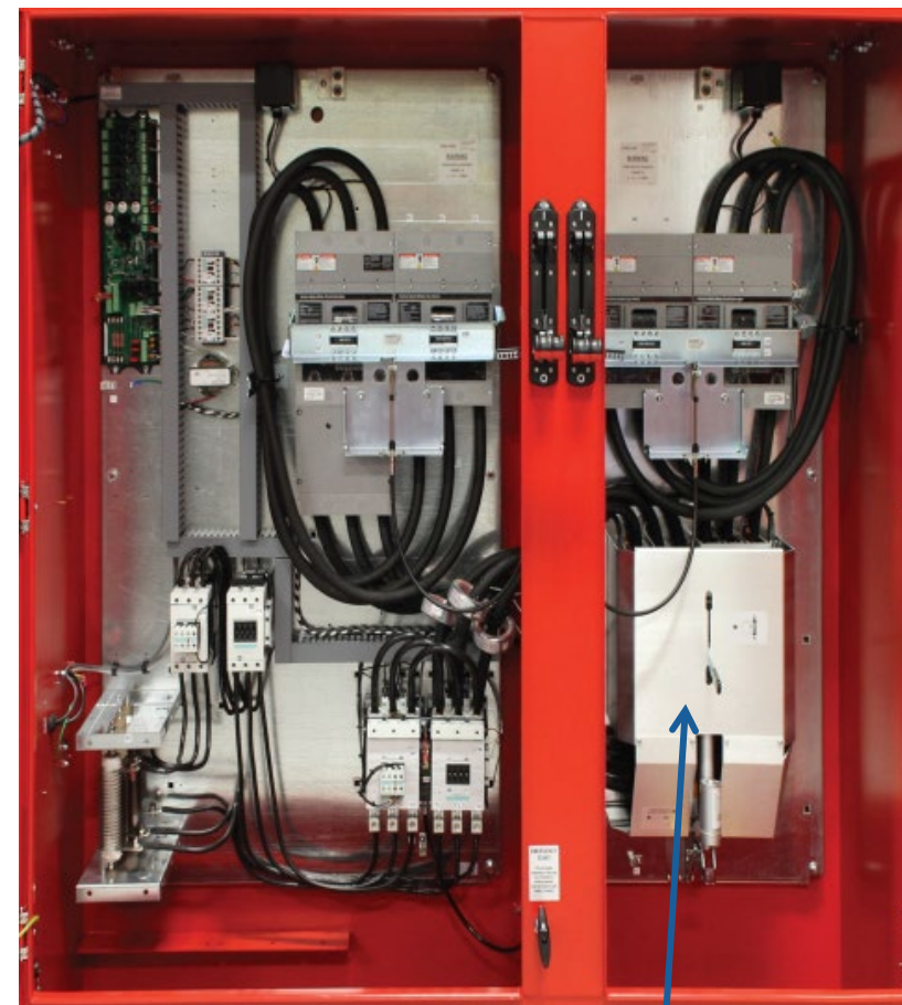
Automatic Transfer Switch
