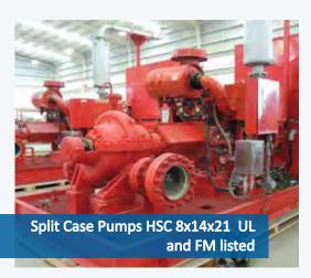
Engineering for the Petroleum & Process Industries (Enppi) has purchased new Fire Package Systems consisting of two split case pumps, model HSC 8x14x21, driven by a 382 HP diesel engine.
